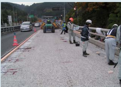
(床版切削状況)
