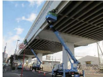
Example of bridge inspection
