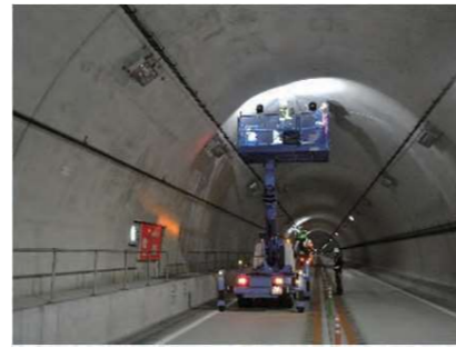
Example of tunnel inspection
