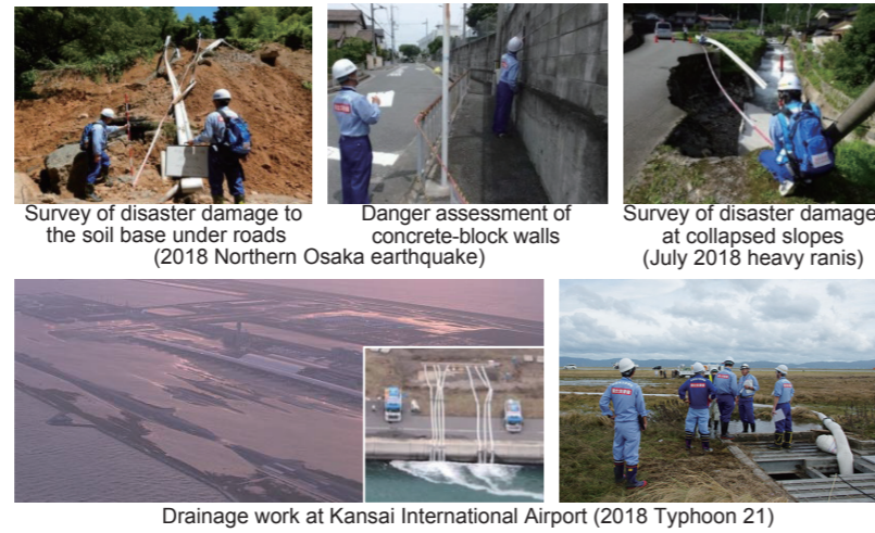
Drainage work at Kansai International Airport (2018 Typhoon 21)
