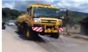
Removal of sediment deposited on road surfaces (2017 Heavy rain in North Kyushu)
