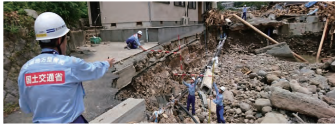
Implementation of investigation of the disaster situation of collapsed roads (2017 Heavy rain in North Kyushu)
