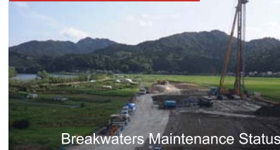
Breakwaters Maintenance Status
