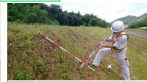
堤防、護岸の点検
