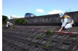
堤防、護岸の点検
