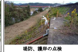
堤防、護岸の点検
